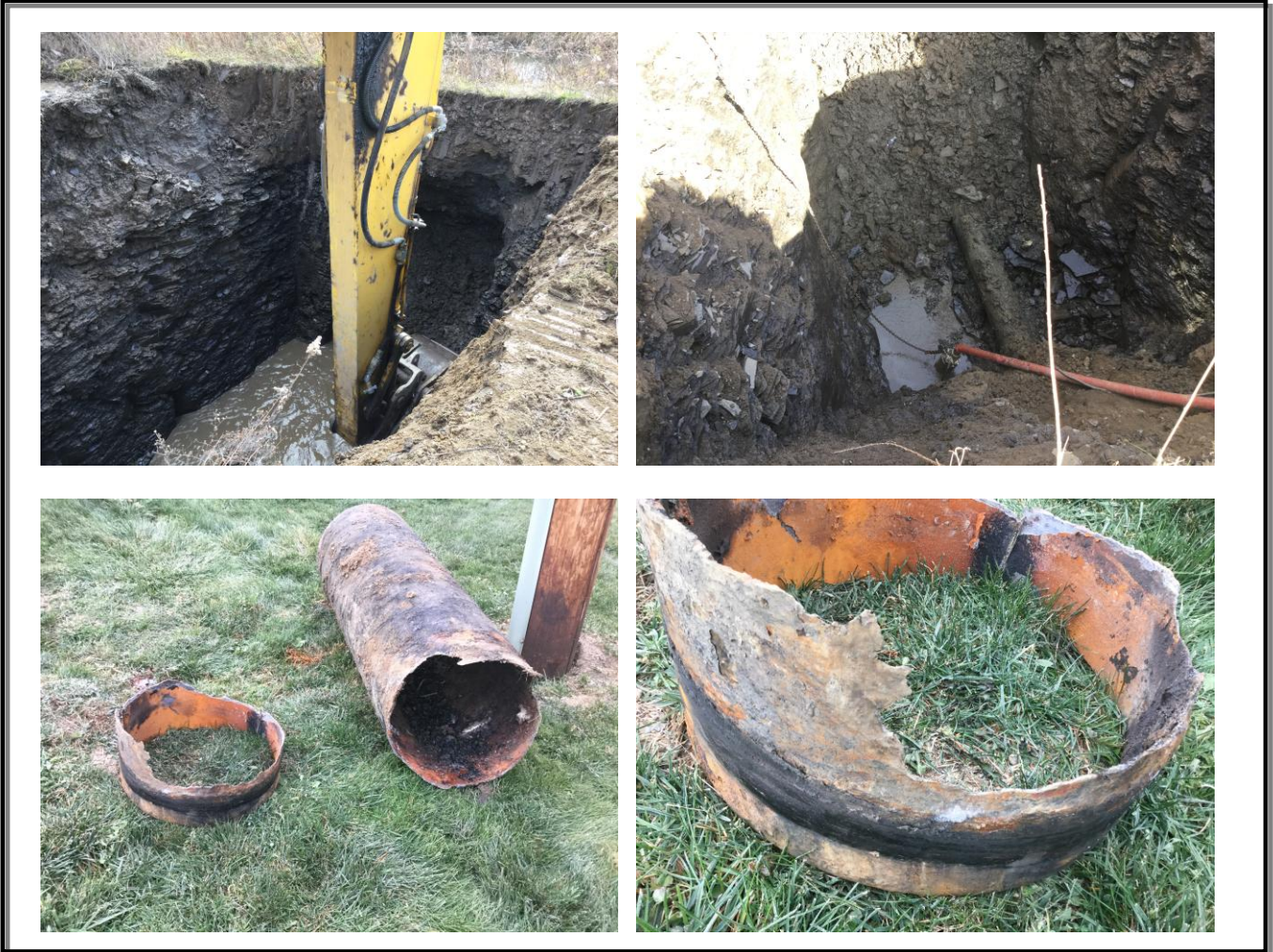
Figure 4: 2016 Construction (MH 37 – MH 38)
