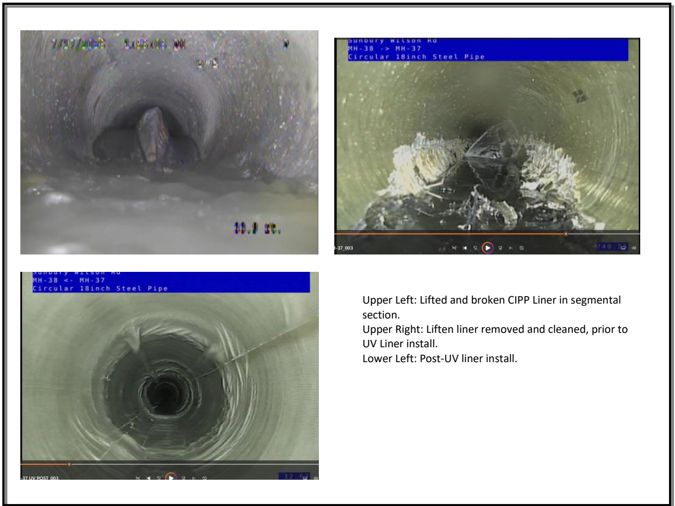
Figure 8: 2025/2026 Lifted liner and UV liner Rehabilitation (manhole 37 - 38)
