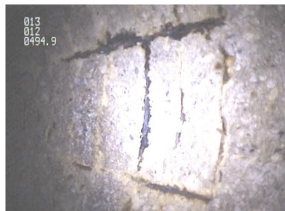
Exposed Rebar Cages
