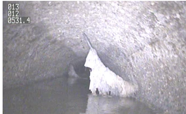
Defective Gaskets
