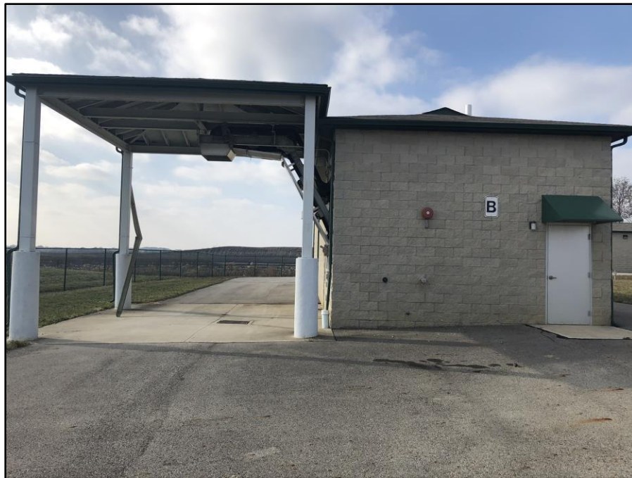
Figure 2-15: Dewatering Building Unloading Area
