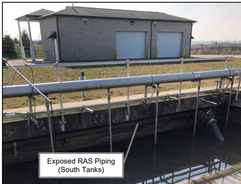
Figure 2-6. Exposed RAS Piping
