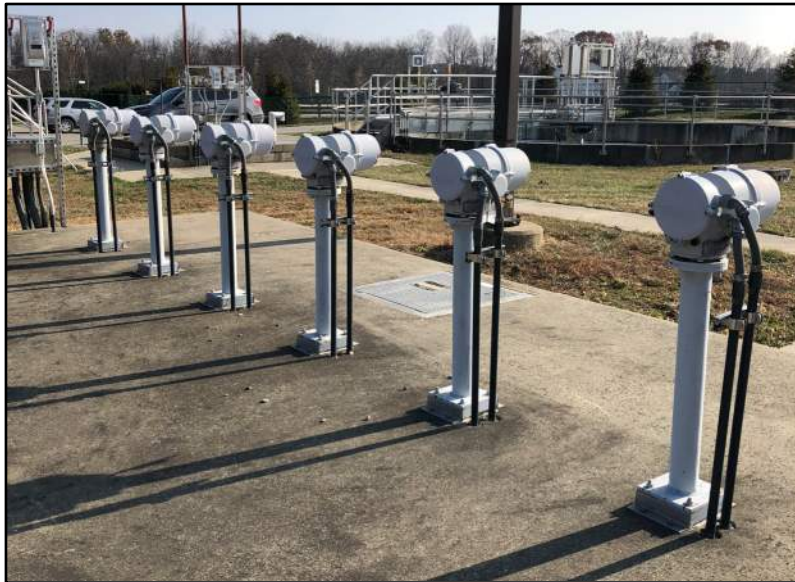
Figure 2-8. RAS / WAS Valve Actuators
