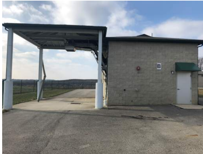
Figure 5-5. Dewatering Building Unloading Area
