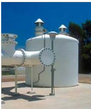
Figure 3-2 Typical Activated Carbon Tower
