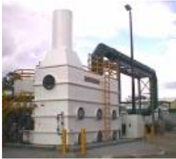
Figure 3-1 Typical Wet Scrubber
