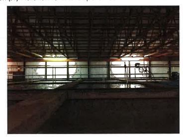
This photograph provided above illustrates the impact of normal typical daily morning flows on the Aeration Tanks 2 and 3. This photo shows less than six (6) inches of freeboard currently available. Normal design practice allows for at least 18-24 inches of freeboard under all peak flow conditions.
